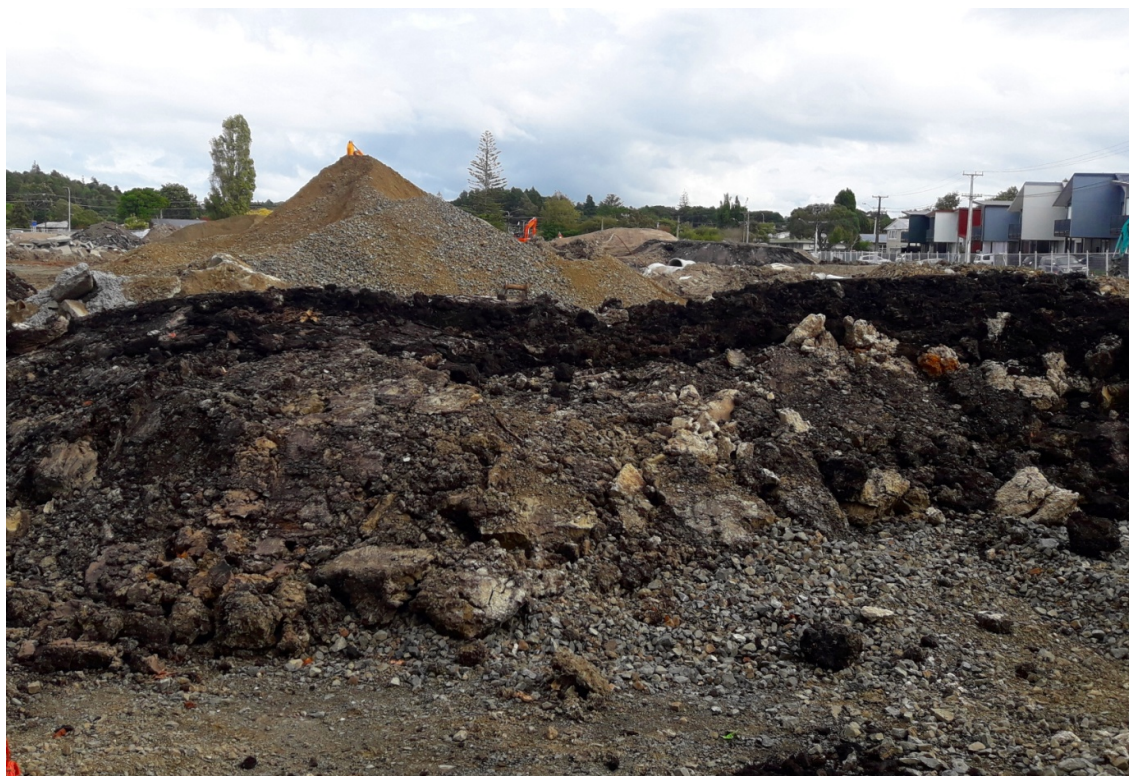
Figure 35: Peat excavated next to stage 3Dii/4A.
